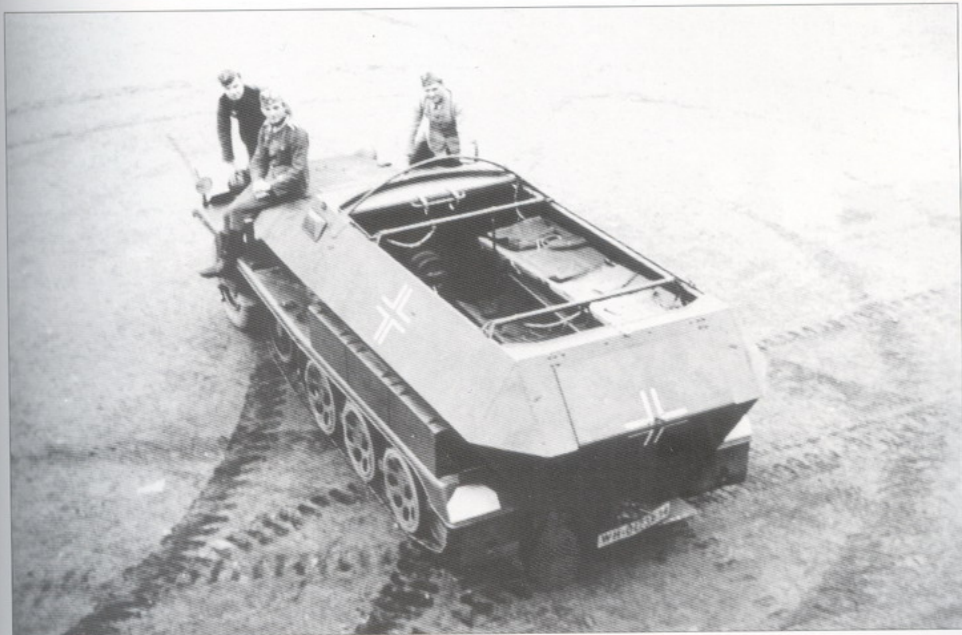
An Sd.Kfz.251/8 Ausf.C (mittlerer Sanitätswagen) unarmed ambulance. It could carry either 4 wounded on stretchers or 8 lightly wounded soldiers.
