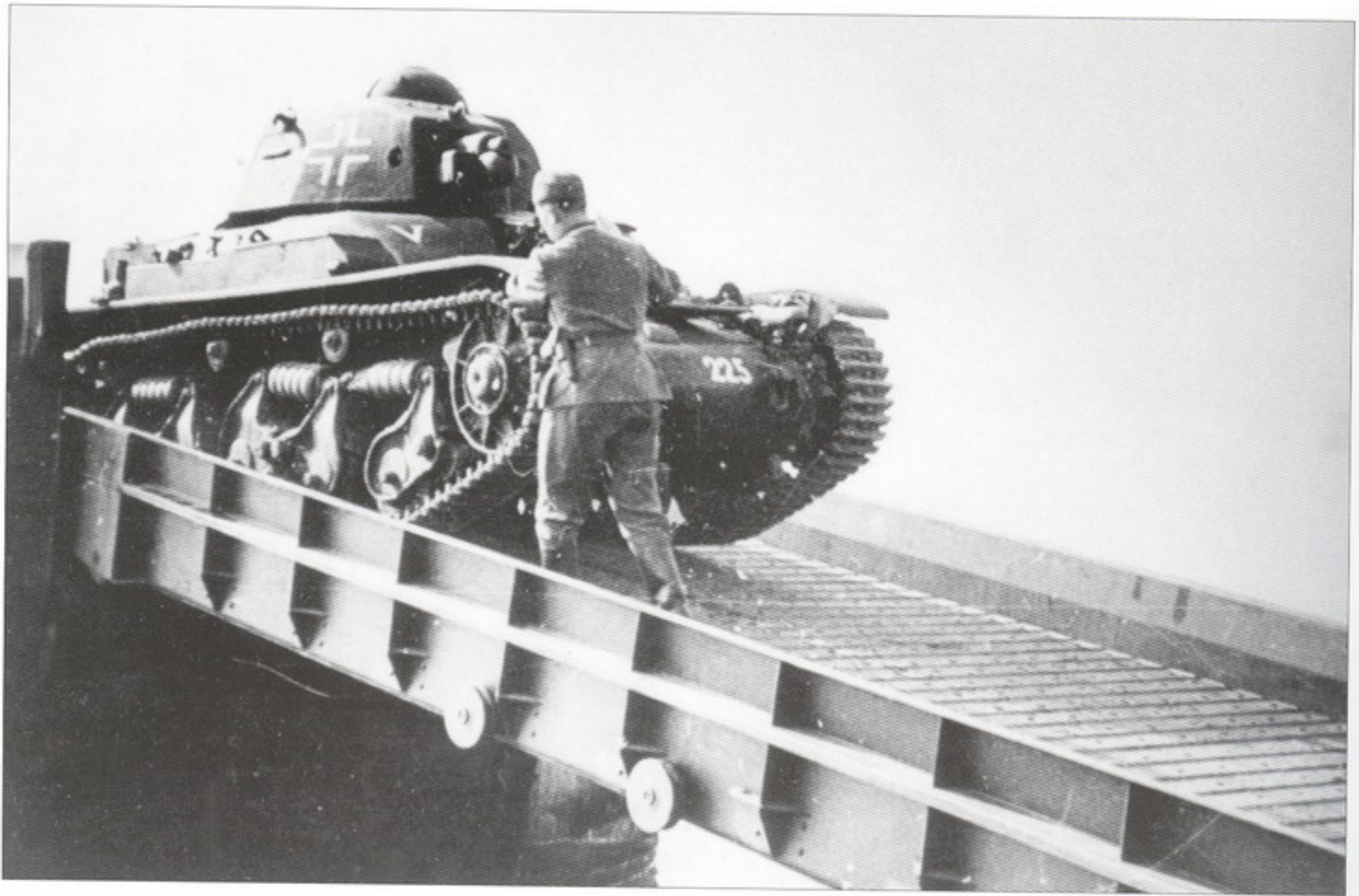
Details of an unloading ramp of an unidentified barge planned to be used for Operation Sea Lion.
