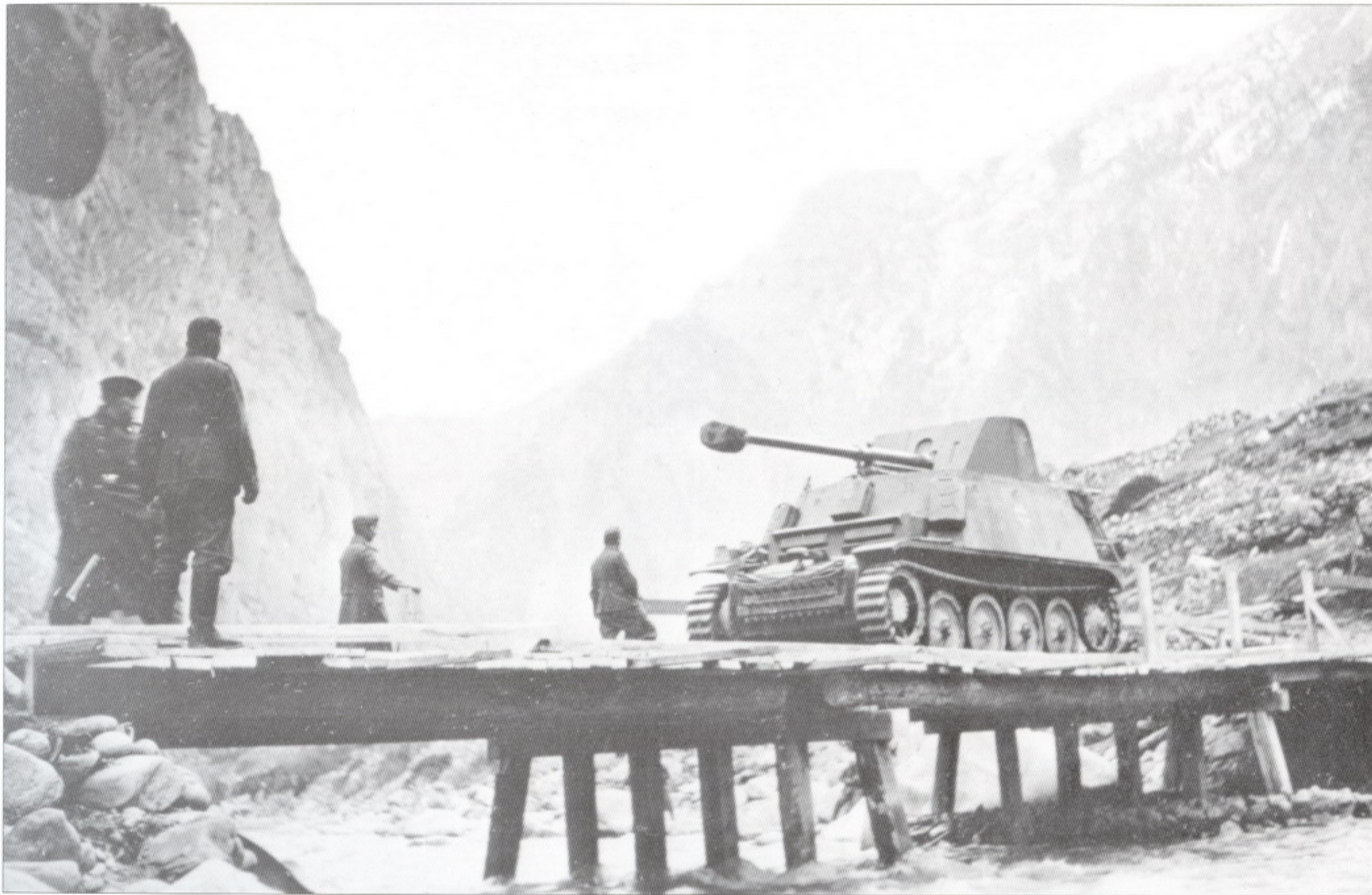
An Sd.Kfz.132 Marder II armed with a 7.62 cm Pak(r) , built on a Pz.Kpfw.II Ausf.D (or E ) chassis, testing the carrying capacity of a bridge built by German engineers in the Kuban in 1942.
