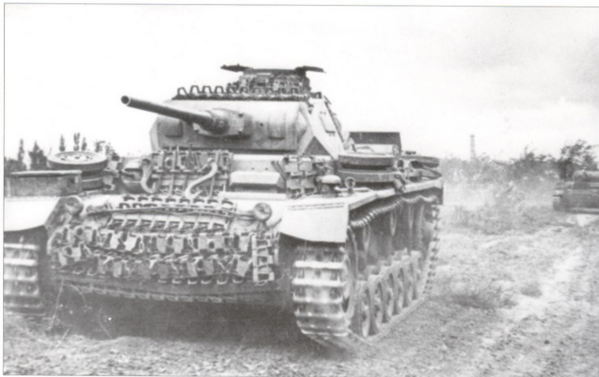
An often-seen field modification on German tanks were extra track links mounted on the front of the hull and superstructure for added protection of the crew. On this Pz.Kpfw.III Ausf.L the extra track links have also been added on the side to protect the gunner and driver.
