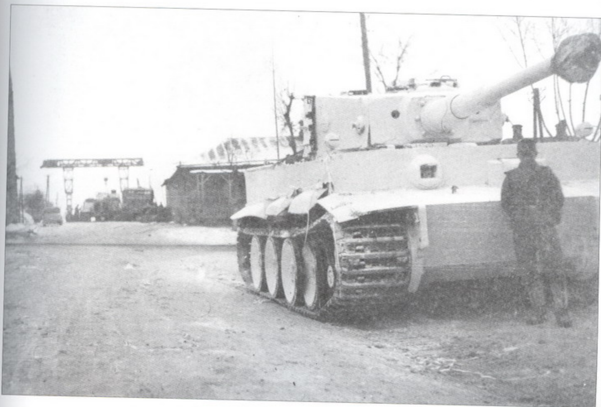
A Tiger on the Eastern Front being repaired and after repairs by the Werkstatt company. Serious repairs of Tigers and Panthers (especially when working on the turret) required the use of the " Fries " 16 ton portable crane.
