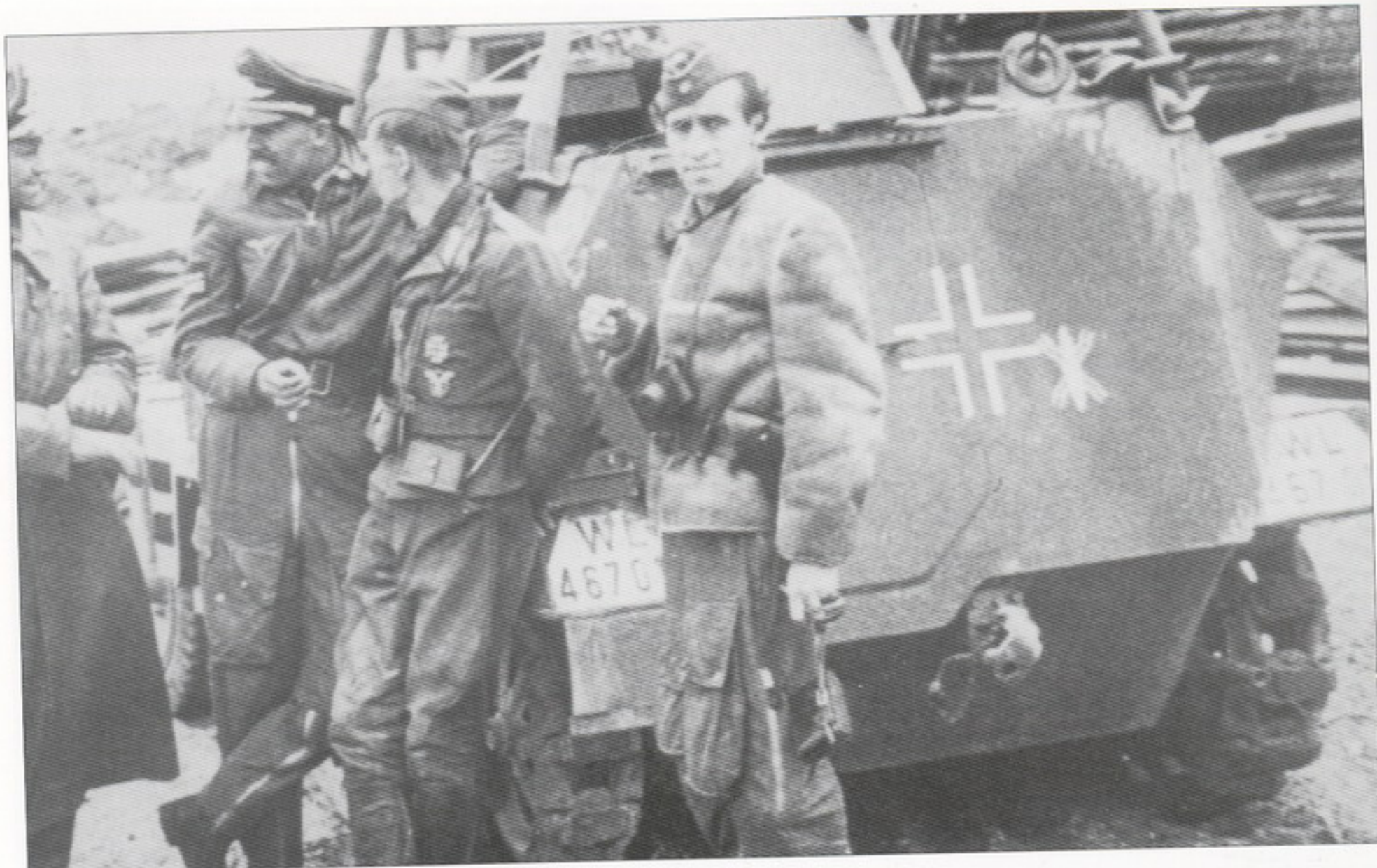
An Sd.kfz.250/3 (Funkwagen), note that it has a gun shield installed on the rear machinegun (usually the shield was installed on the forward MG 34). Also of interest is the unit insignia (next to the Balkenkreuz). It is probably from the Bordfunkerschule, as this insignia has also been seen on a Ju 52/3m which was used to train radio operators for the Luftwaffe.
