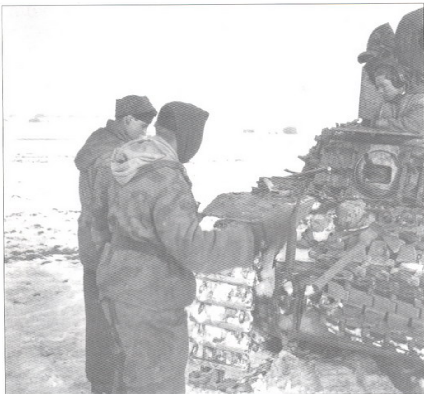
A Pz.Kpfw.IV Ausf.H , number 546 of Feldwebel Rudl, after an attack from an IL-2 Sturmovik. Its crew is fixing the damaged track on the banks of the river Styr, near Lutsk, January 1944.
