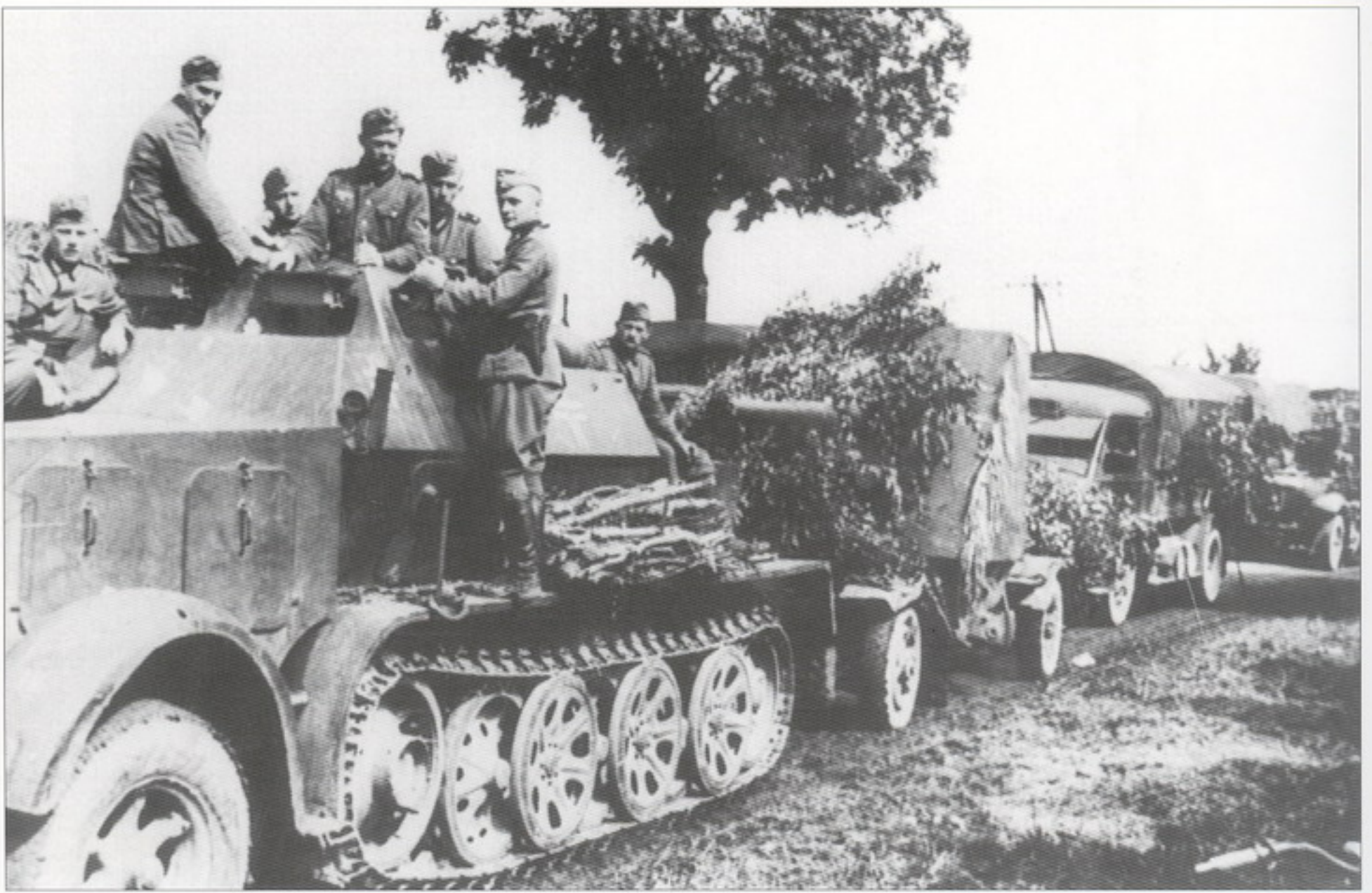
An Sd.Kfz.7 with a partially armored superstructure serving as a prime mover for a special version (socalled Bunkerflak) of an 8.8 cm Flak . The Flak has an enlarged gun shield installed.
