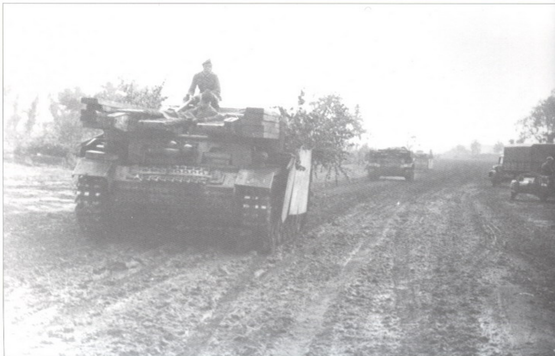
A group of Pz.Kpfw.III Ausf.L tanks ( Bergepanzer ). The one in the foreground is transporting elements for building an engineer bridge.
