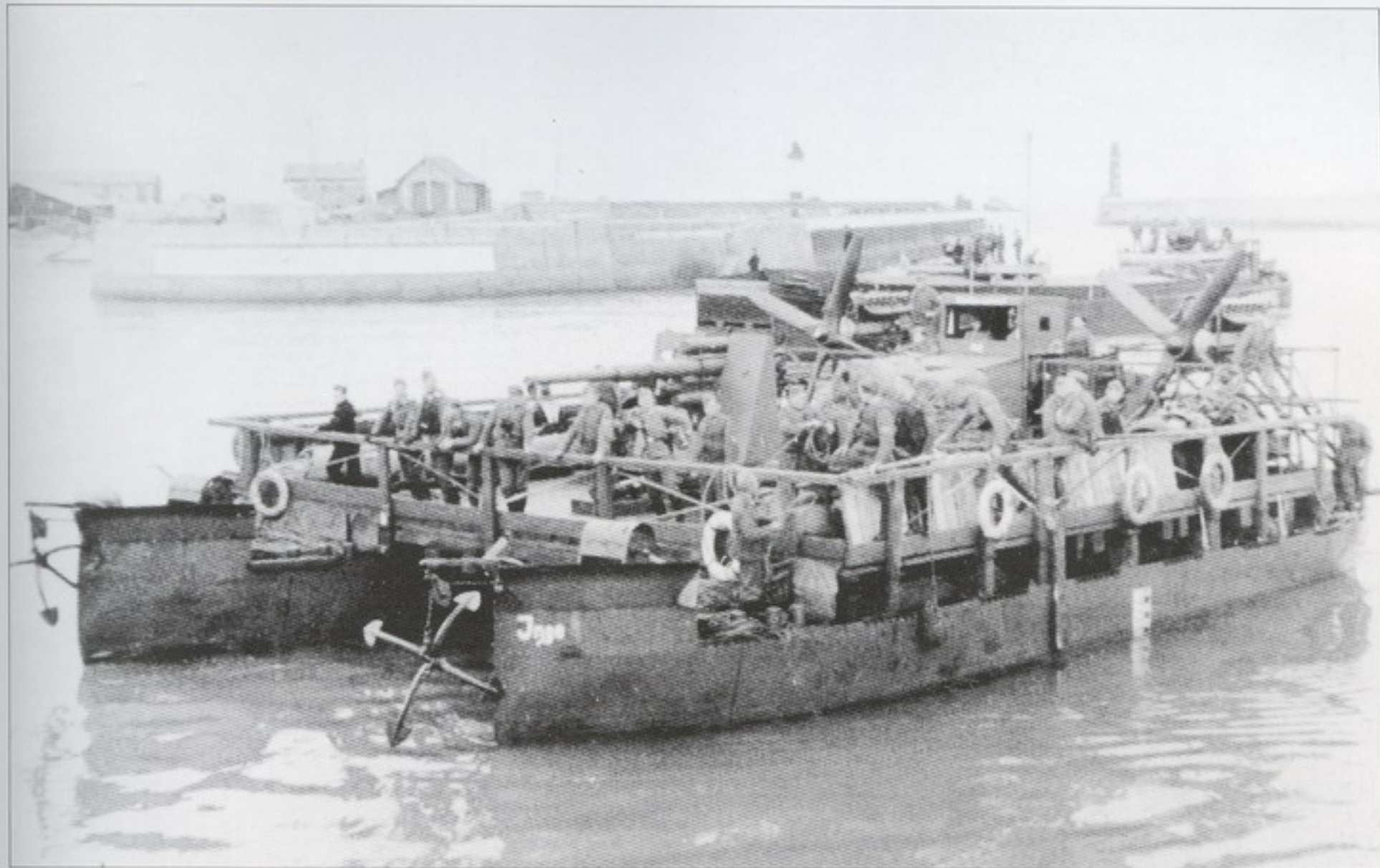
The Herbert-Fähre ferry (expedient transport for Operation Sea Lion) was built on the basis of ex-Austrian material for bridge building and had a temporary wooden deck. There were 14 such transports built. The prototype was built by Pi.Btl.47 (Engineer Battalion) and was powered by 2 BMW VM airplane engines (660 HP, four-bladed propellers) and three Ford V8 engines (78 HP, directed through u-joints to propellers). Its armament was an 8.8 cm Flak 18 gun and it had a carrying capacity of 35, 000 Kg. This ferry was photographed in port Fecamps in 1940.
