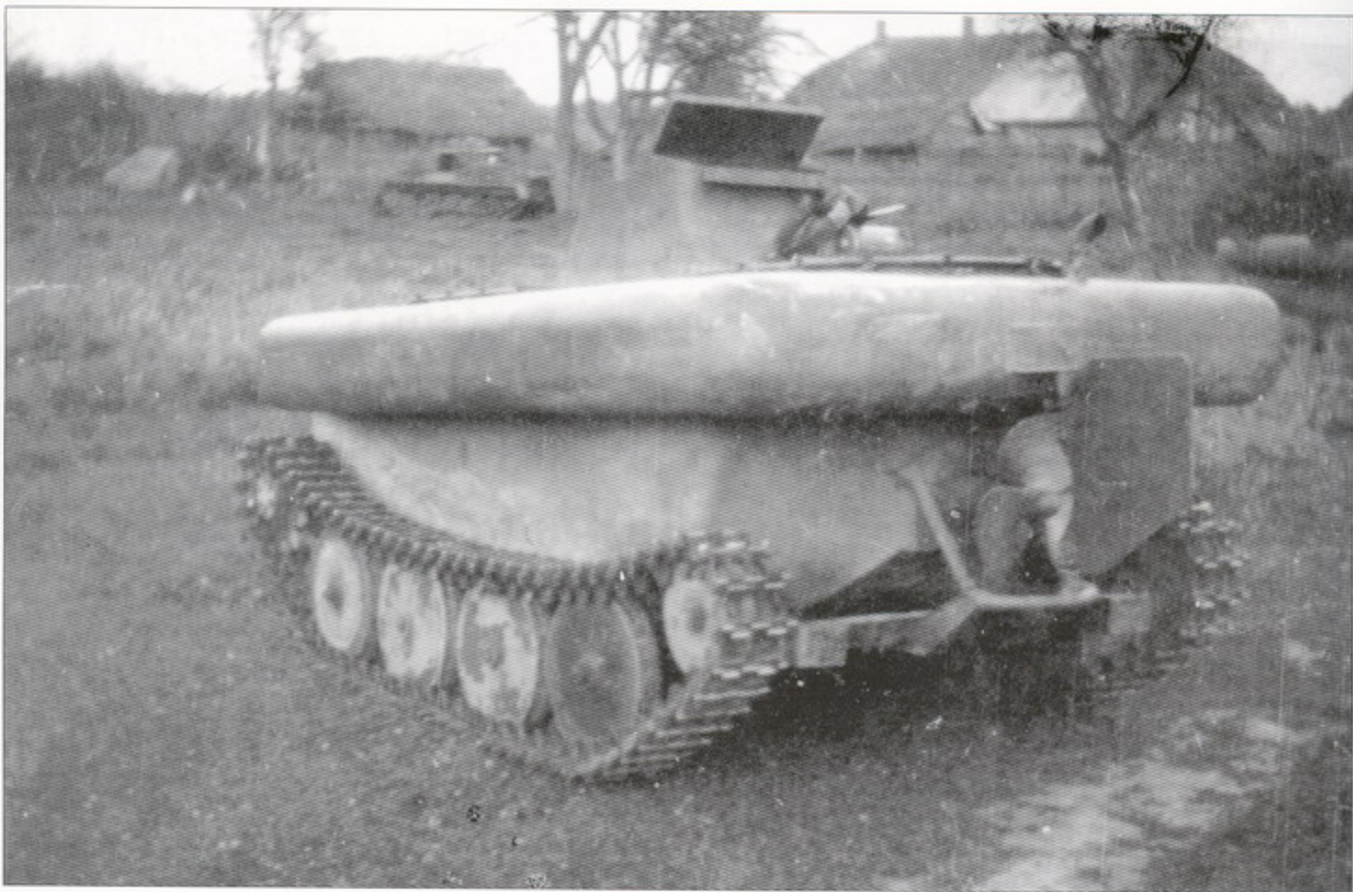
The Ente (Duck), a small amphibious tank, steered in a similar fashion to the Goliath ( Ladungstrager ), was a vehicle which carried an explosive charge. These two vehicles belong to Pi.Lehr.Btl.1 and were photographed in the autumn of 1941 in the Wolchow region of the Northern part of the Eastern front.
