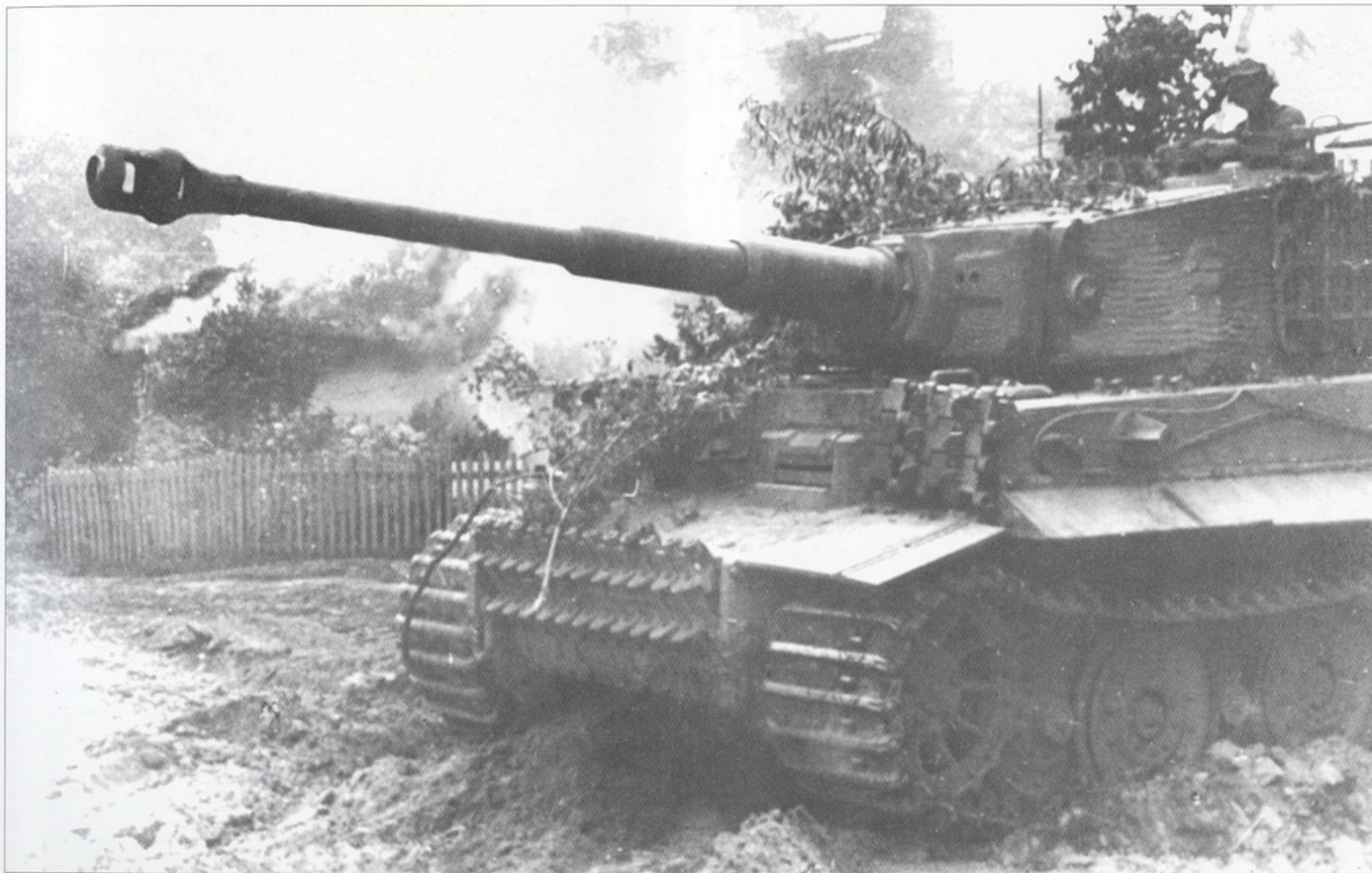
A late production Tiger I with steel road wheels. Taken on the Eastern Front in the summer of 1944, this is a very interesting photo as it confirms information which claims that a type of active armor (made up of screening plates) was used on German tanks in combat. These plates were also tested on the Panther. Photos of a Panther found in Poland show identical fittings to those seen in this photograph, located at the front of the hull adjacent to the driver's station.
