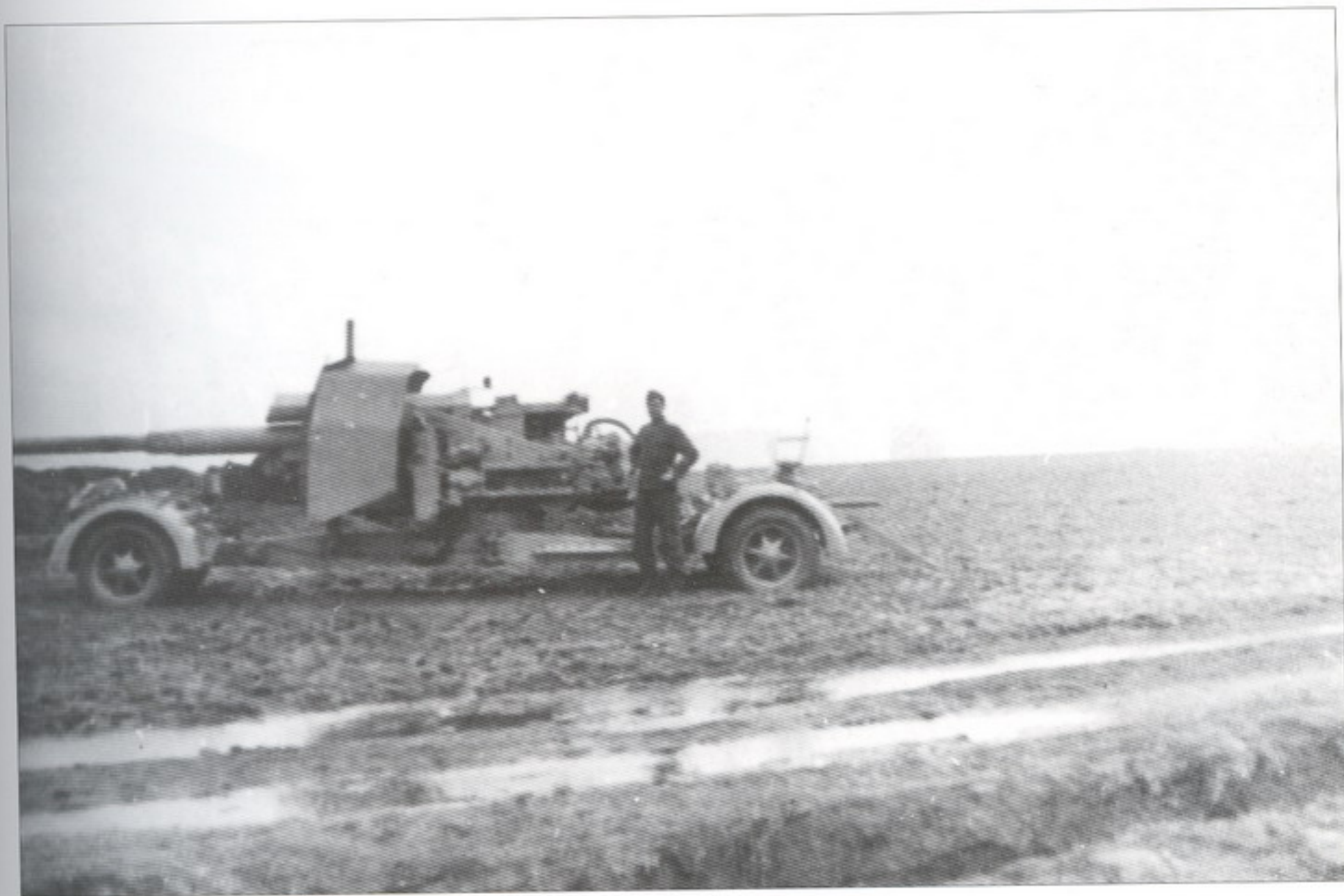
The 8.8 cm Pak 43 , with its L/71 gun barrel, was the last version of the 8.8 cm gun. It had no equal when it came to destroying enemy armor at long distances. This one has 2 victories marked.
