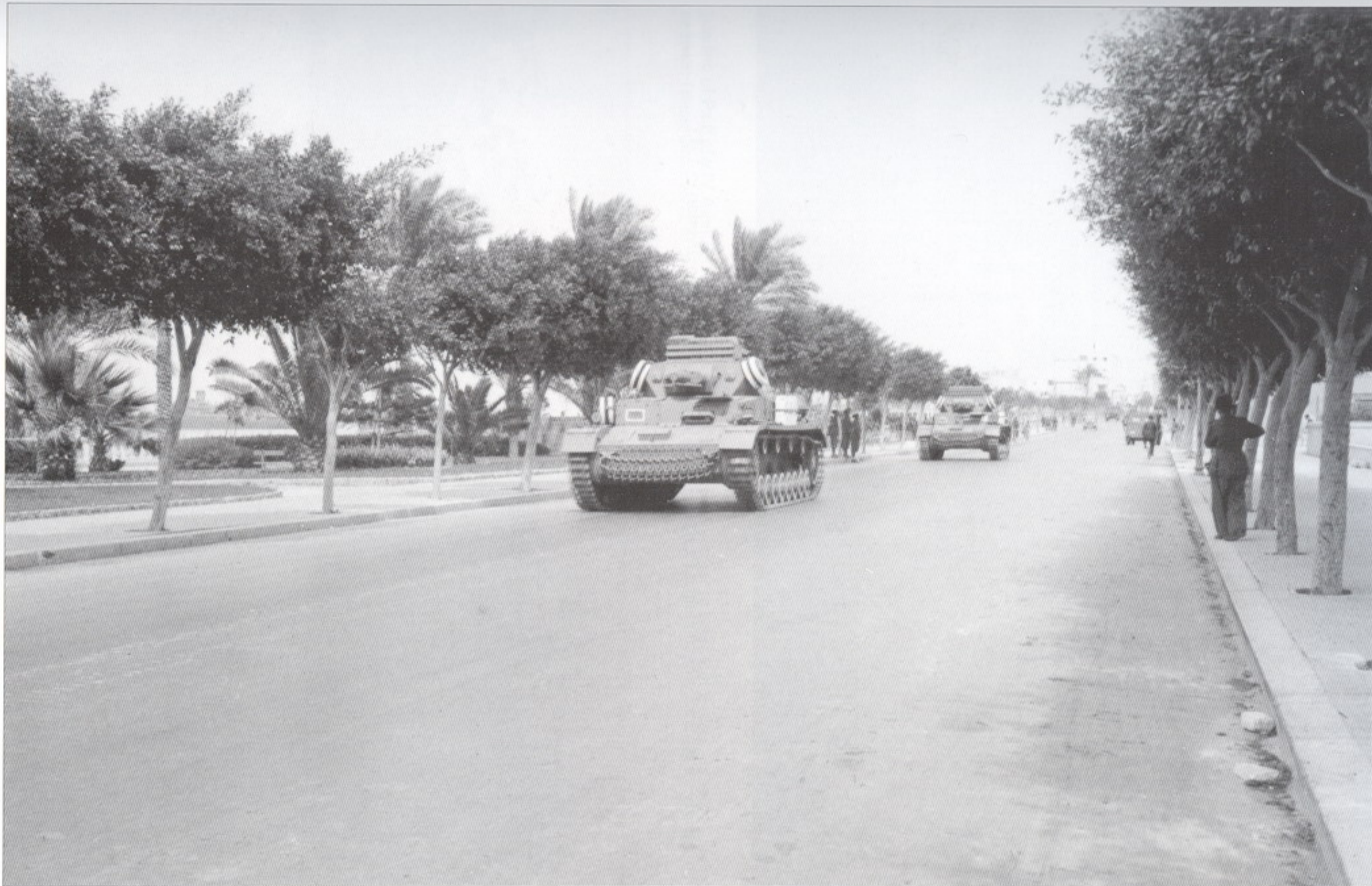
Pz.Kpfw.IV Ausf.E tanks of the 15. Panzer Division, "Deutsches Afrika Korps". To prevent excessive heating, the rubber rims of the road wheels were painted white. The water canisters were also painted white.
